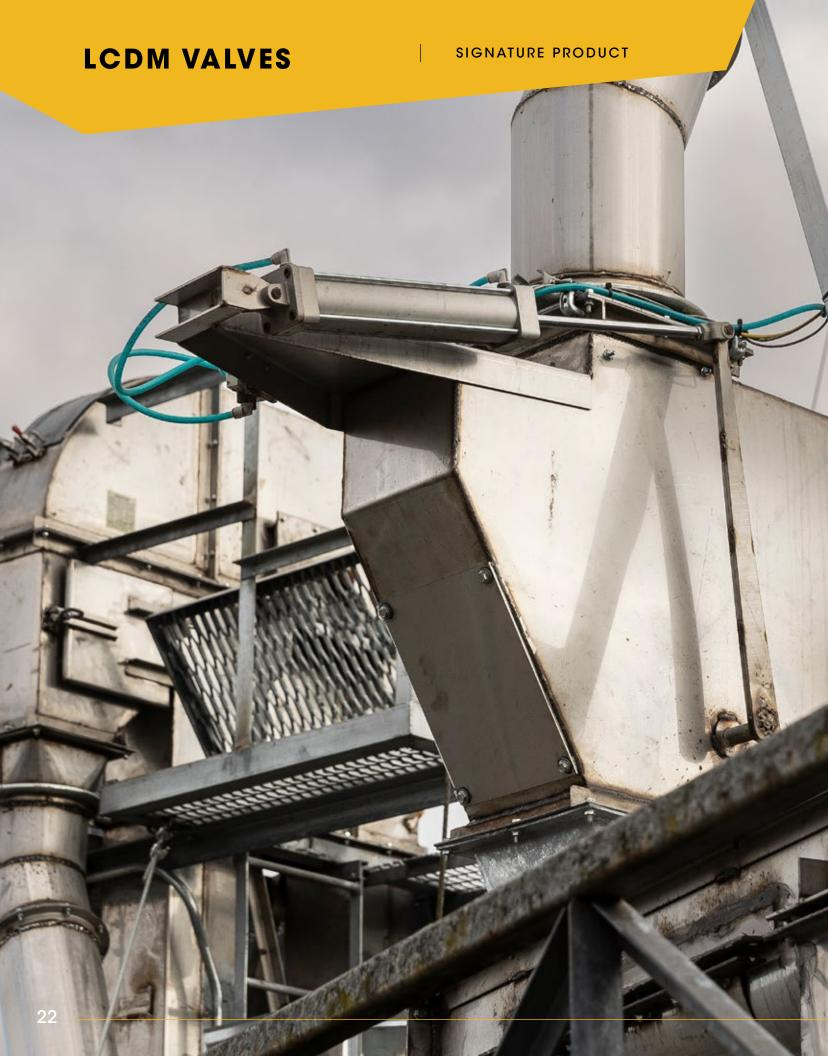
LCDM Valves are unique in that they are "full flow". What does this mean? Many of the valve designs in the industry today restrict the flow of grain. For example, an 8" valve will not effectively handle the capacity of the spout feeding it. However, LCDM Full Flow Valve's were designed to handle this capacity without having any restriction of flow. This means that you can fully accommodate the flow from the spout and maximize the flow of grain when the valve is open.
