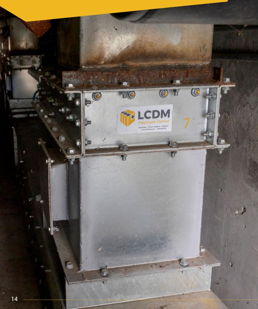
LCDM Slide Gates are uniquely designed to meet your needs, maximize efficiency and offer best in class reliability. Our slide gates make controlling the flow of grain and other bulk materials at discharge points easy. With several options to choose from, LCDM can accommodate all your grain flow requirements.
