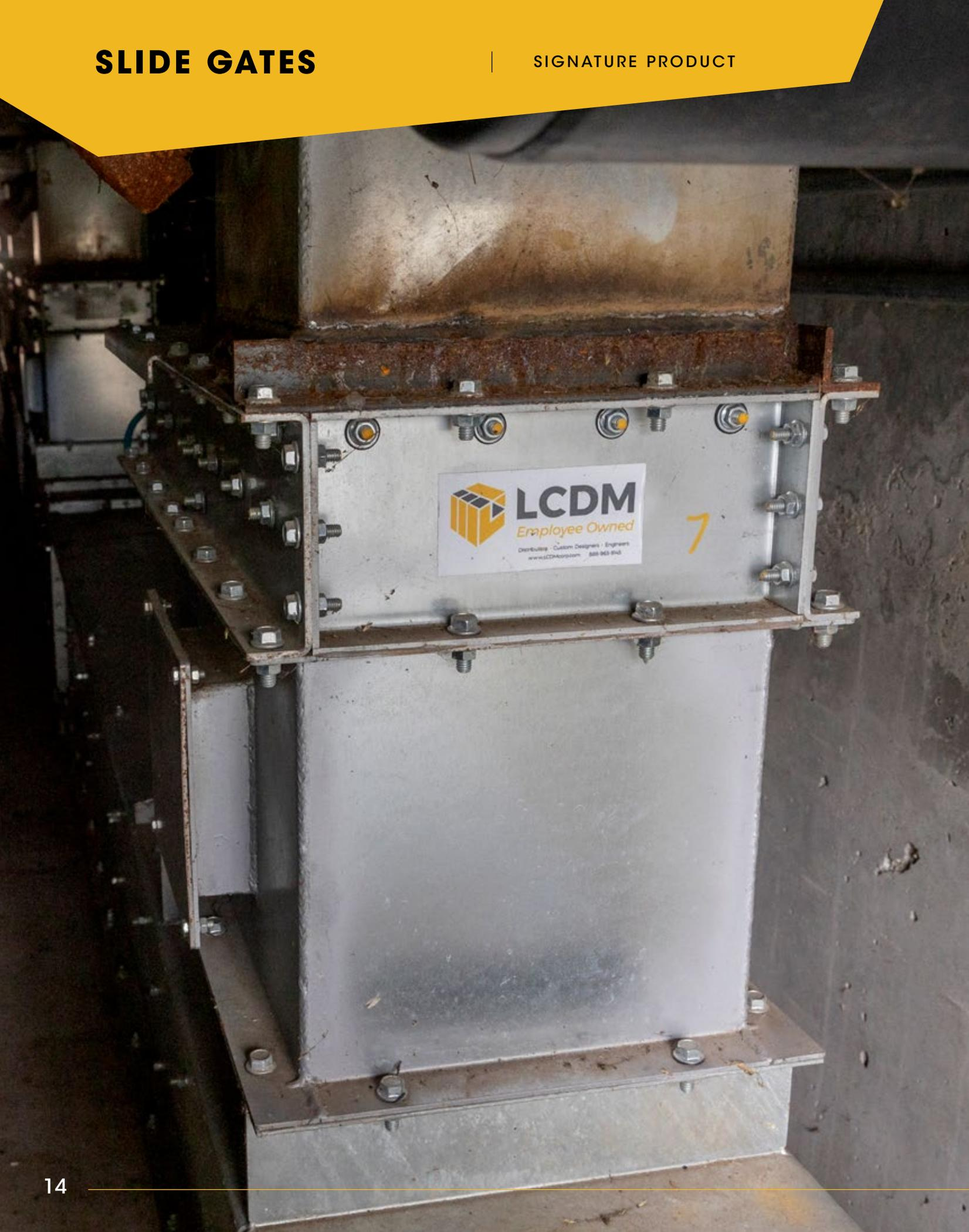
LCDM Slide Gates are uniquely designed to meet your needs, maximize efficiency and offer best in class reliability. Our slide gates make controlling the flow of grain and other bulk materials at discharge points easy. With several options to choose from, LCDM can accommodate all your grain flow requirements.
